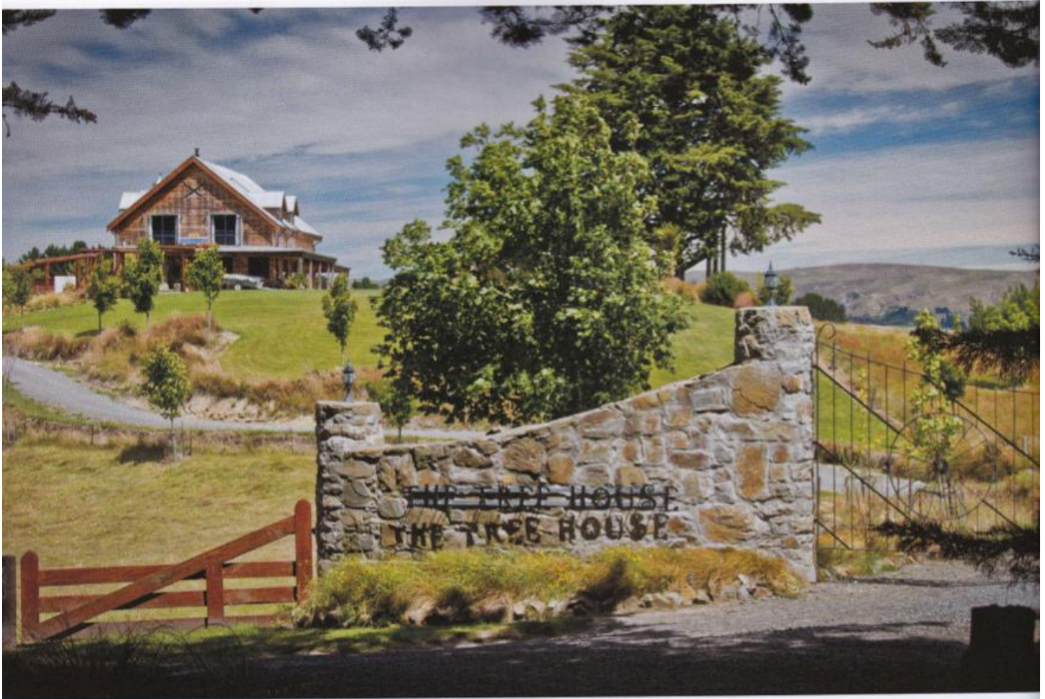
Entrance to The Tree House.
